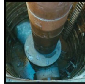
Fig. #3: 120" ID to 78" ID Tunnel Shaft
